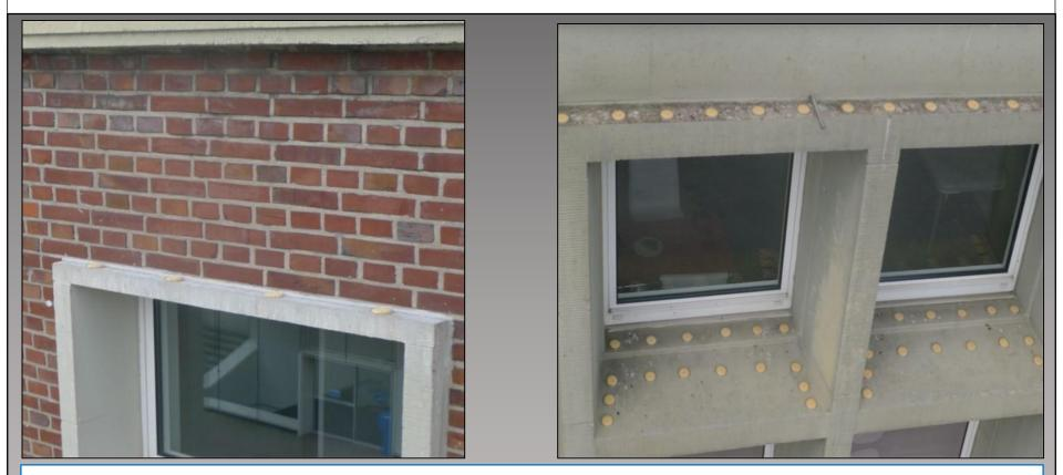
Being a listed building, the local heritage officer would not agree to the use of spikes, wires or nets, while the client wanted a permanent, unobtrusive solution. The building was cleaned of droppings, and 小島 *Bird Free* was installed.
